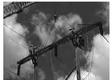
8 Crane raises arm to new location
