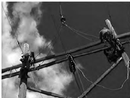
7 Crane cable is attached to crossarm. Double arm assembly is spread apart at each pole using hydraulic jacks. Crossarm bolts are removed.
