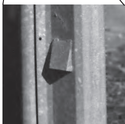
Available covered vent hole reduces moisture build-up inside cover.
