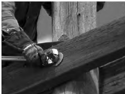
4 Loosen crossarm mounting hardware but do not remove.
