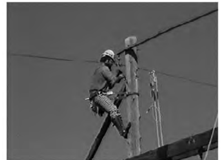
3 Unbolt existing knee braces (if applicable)
