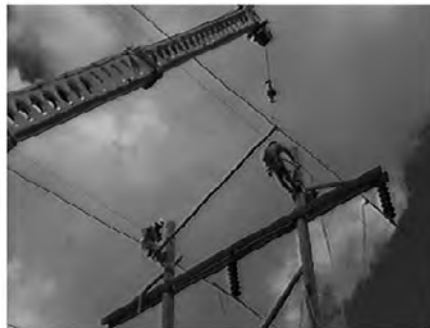
5 Top steel angle removed and lowered to the ground
