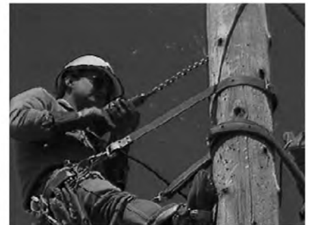
6 Drill poles for new bayonets and crossarms
