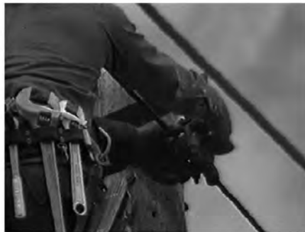
2 Disassemble shield wire attachments from top of pole
