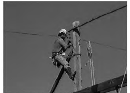
3 Unbolt existing knee braces (if applicable)
