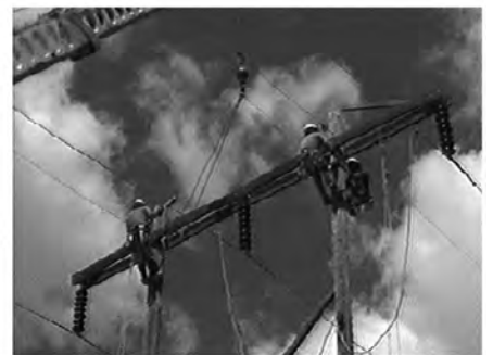
8 Crane raises arm to new location
