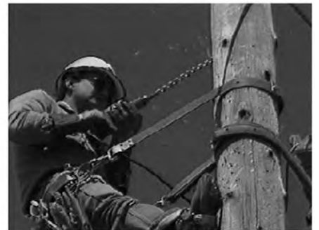
6 Drill poles for new bayonets and crossarms
