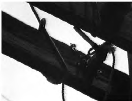
7 Crane cable is attached to crossarm. Double arm assembly is spread apart at each pole using hydraulic jacks. Crossarm bolts are removed.
