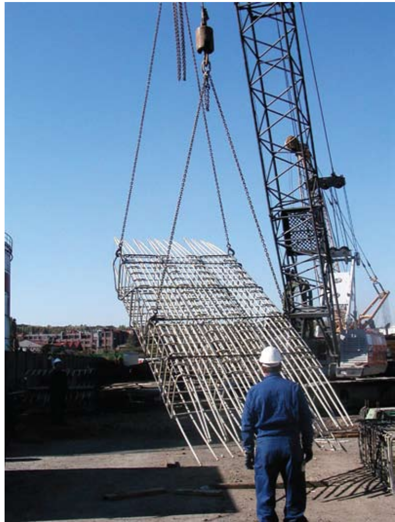
Lifting cage using a temporary support frame.
