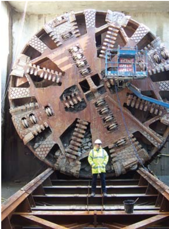
Channel Tunnel Rail Link London ENGLAND
