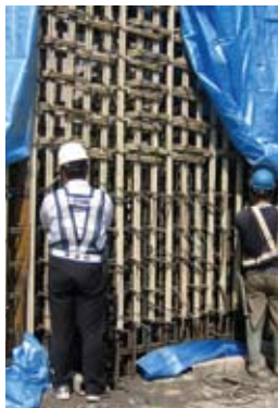
Lifting cage using a temporary support frame.
