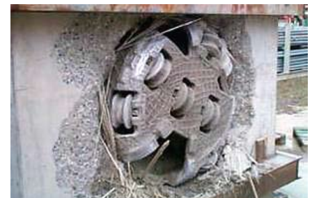
Trial Test Breakthrough at Herrenknecht Factory, Germany
