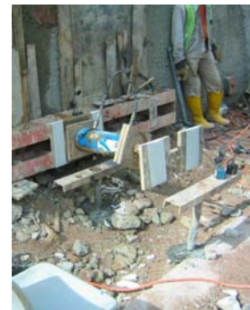
Site Pull-out Test
