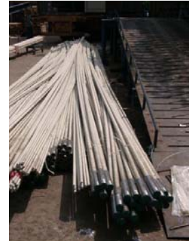
GFRP Soil Nails
