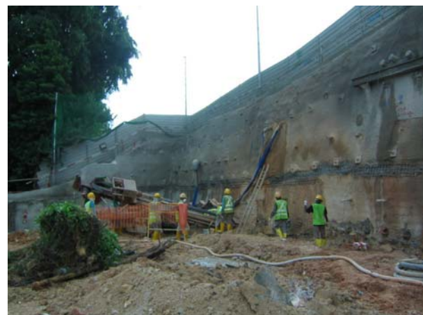
Installation of GFRP Soil Nail
