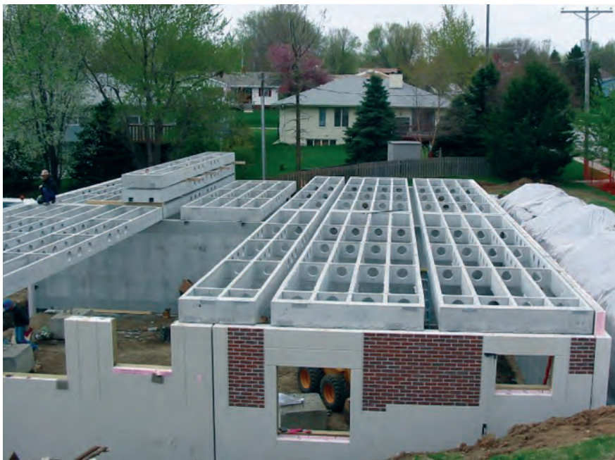
Fig. 17. Completed basement walls with brick finish details and floor panels.
