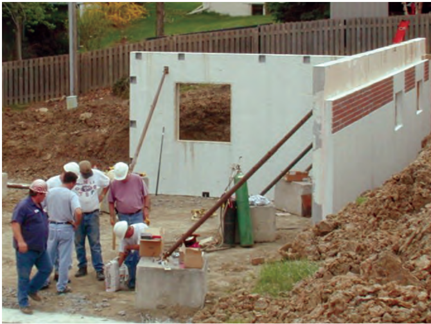
Fig. 16. South end corner walls were the first to be erected.
