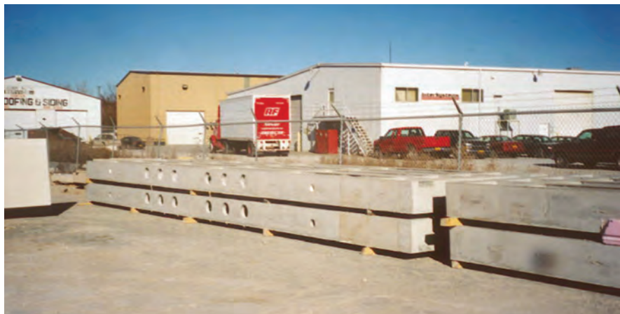
Fig. 9. Side view of concrete floor panels at precasting plant.
