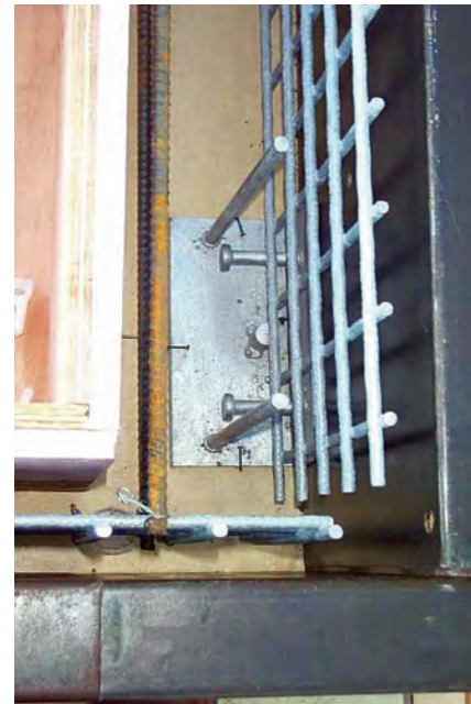
Fig. 8. Special design plate installed in floor panel to be used as a connection to the precast sandwich wall panels.
