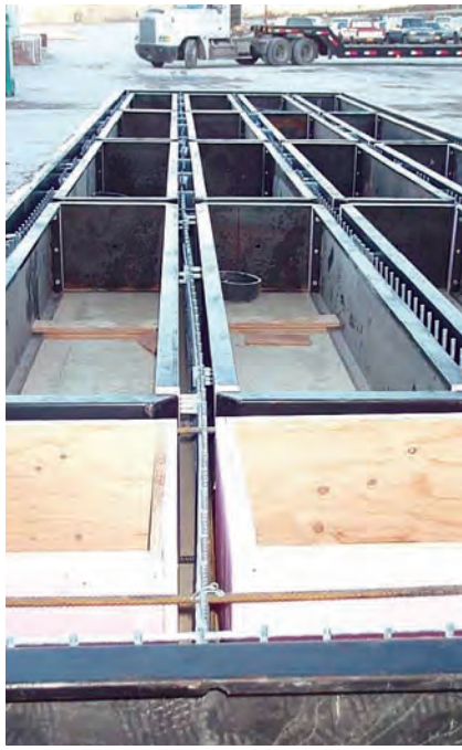
Fig. 6. Formwork and reinforcement of a concrete panel.
