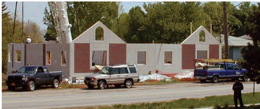
Fig. 20. NU Concrete House following installation of all precast concrete panels.
