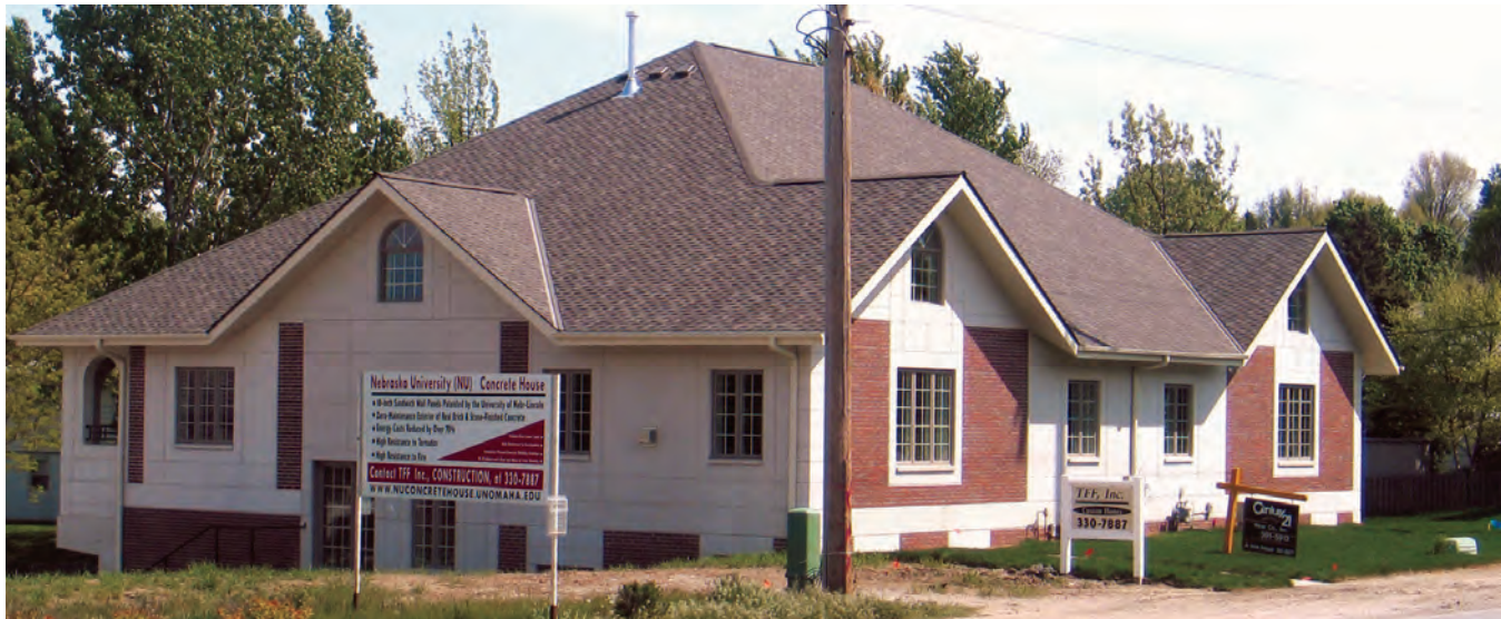
Fig. 1. A precast concrete home demonstration project was built for the first time in the United States in 2003.
