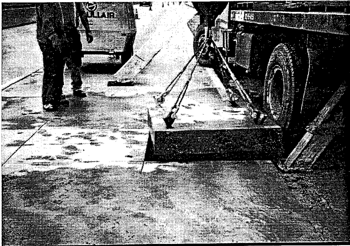
Figure Five Removal of Test Joint Slabs
