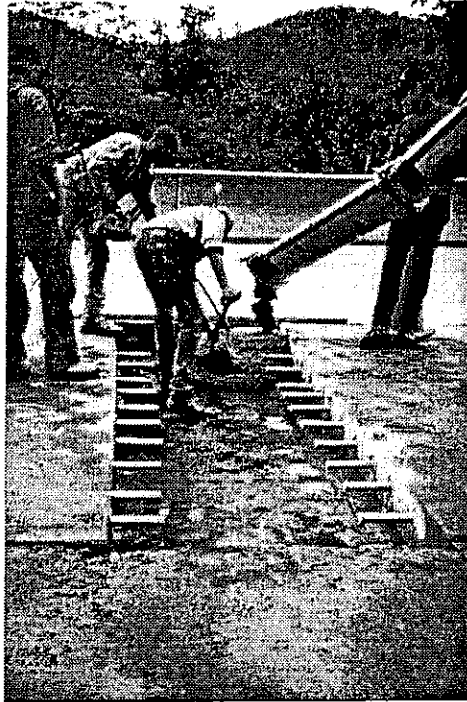
Figure Six Replacing the Test Slab with FRP Composite Dowel Bars
