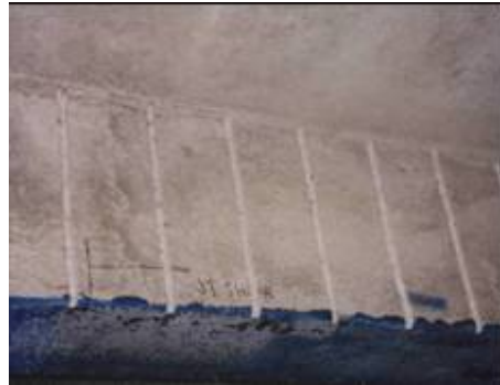
Figure 4 – Shear Strengthening of RC Joist Using Carbon NSM Bars
