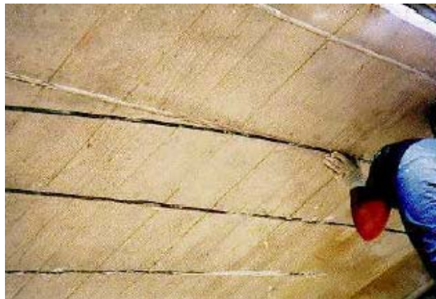
Figure 2 - Strengthening of a Bridge Deck Using NSM Carbon FRP
