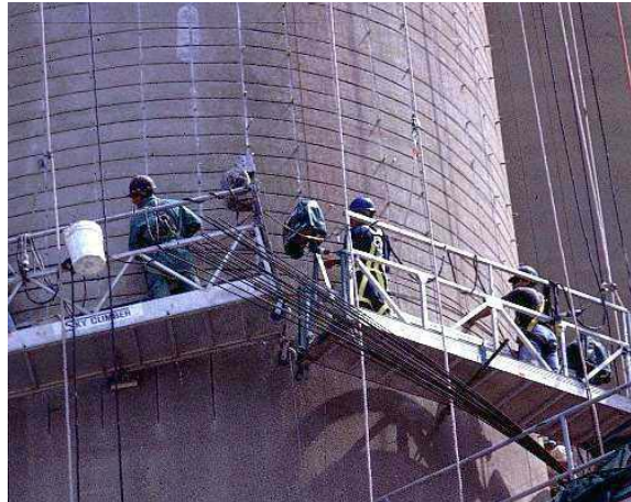
Figure 1 - Strengthening of Cement Silos Using NSM Carbon FRP Bars
