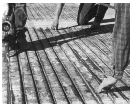
Figure 3 – Negative Moments Regions Strengthening of Bridge Deck with NSM Bars
