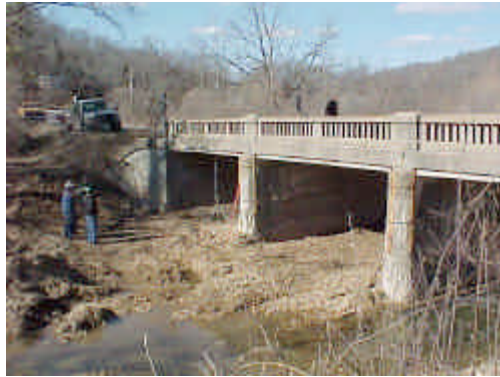
Figure 1 – Martin Spring Bridge
