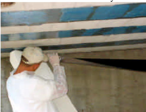
c) Application of CFRP Laminates
