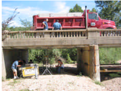
Figure 13 – Load Test with H20 Truck
