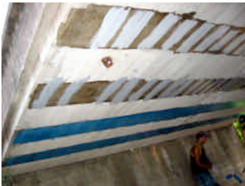
a) Surface Preparation with Primer and Putty
