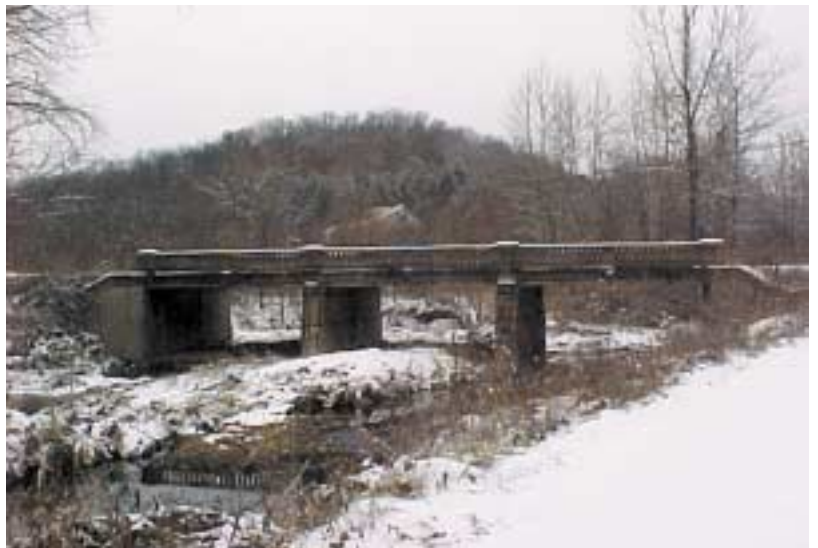
Figure 1: Three-span concrete slab bridge.
