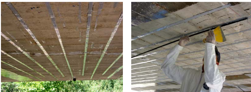
Figure 1 – NSM Installation on a RC Deck Bridge
