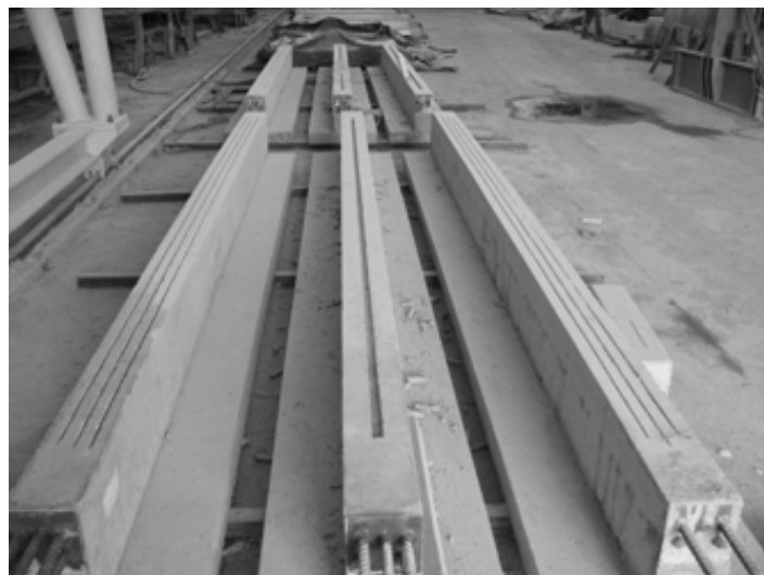
Fig. 3 Details of the slots made at the beams
