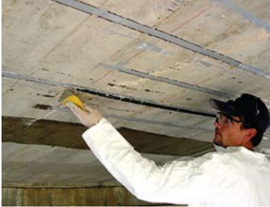
Inserting CFRP Tape on edge.
