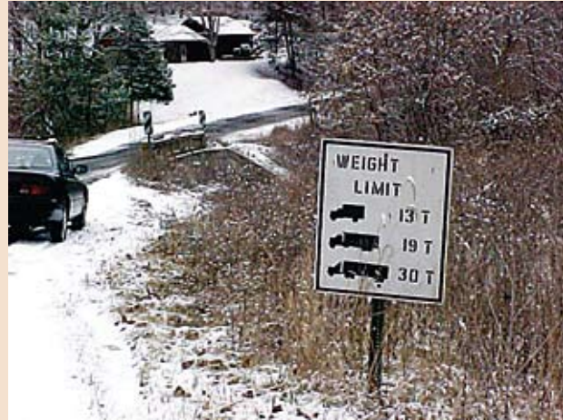
Aslan 500 can be used to remove posted limits on bridges.
