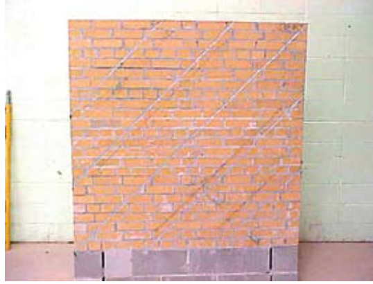
Strengthened installation with clean appearance.
