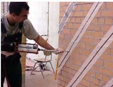
Filling groove with structural adhesive.
