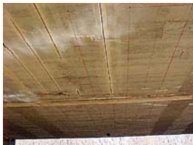
Saw Kerf is cut into element.
