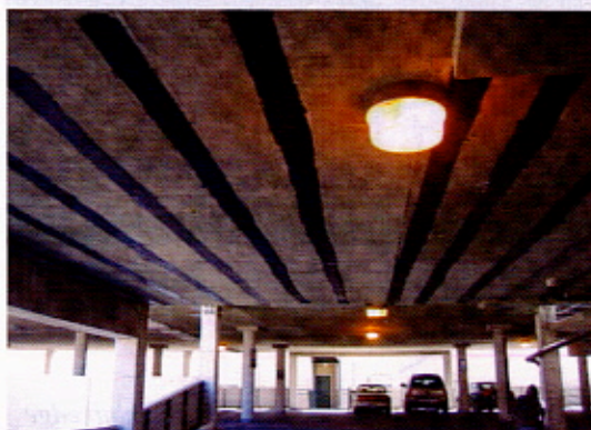
Fig. 3: Slab underside strengthened with CFRP laminates
