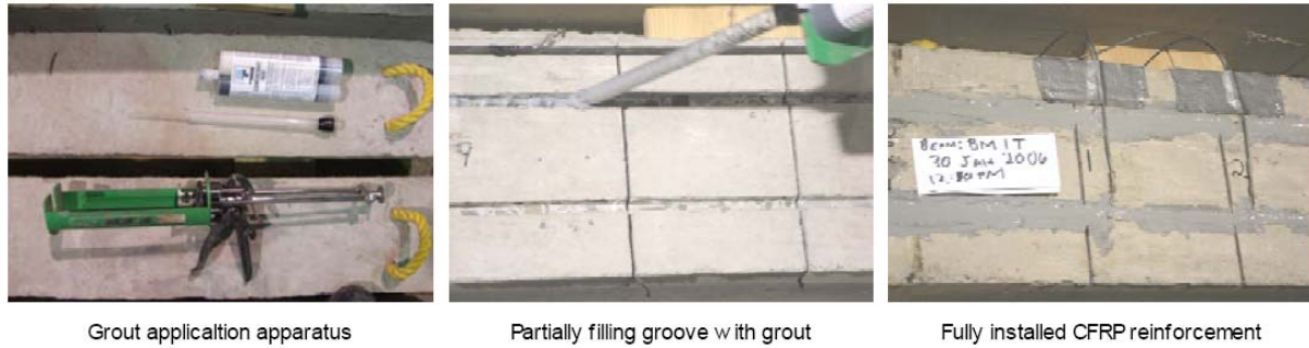
Fig. 4 Installation of CFRP Reinforcement.
