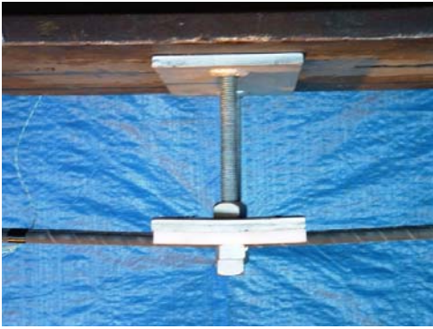
Figure – 5. Photograph of extended deviator with CFRP bars.
