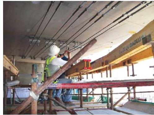
Figure – 2. Trial installation onto soffit of a reinforced concrete slab.
