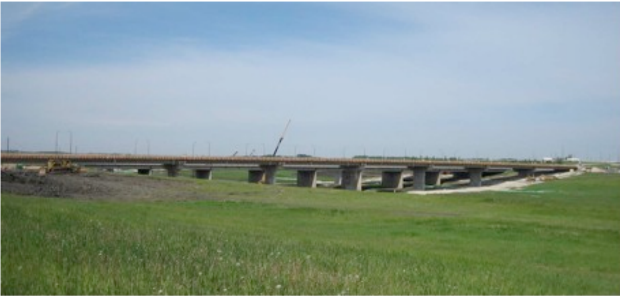
Photo Courtesy of Garth Fallis, Vector Corrosion Technologies
