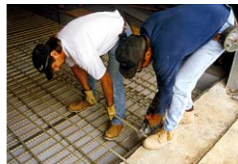
Cutting should be done with fine blade saw, masonry, diamond blade or grinder. Shearing is NOT permitted.
