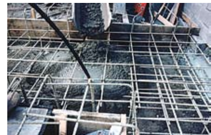
Some bent shapes are made using appropriate lap splicing.
