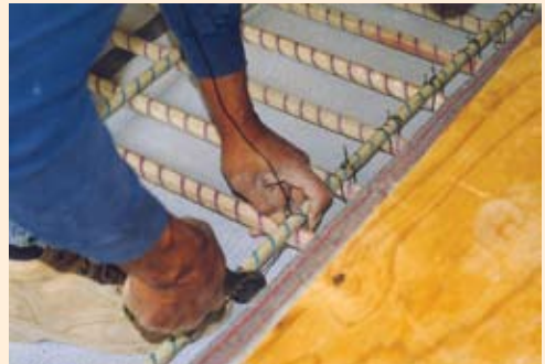
Plastic coated wire ties are recommended. Nylon zip-ties may be used for completely non-magnetic applications.
