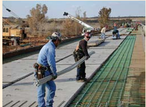
Light weight of GFRP rebar aids installation.
