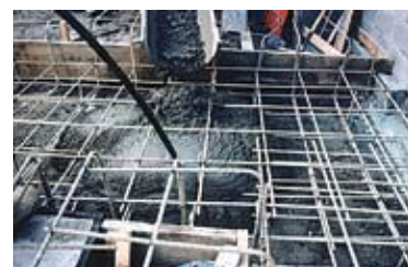
Some bent shapes are made using appropriate lap splicing.
