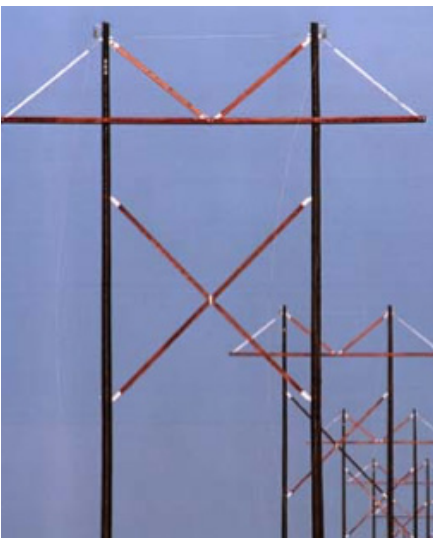
Wood framing up to 345kv
